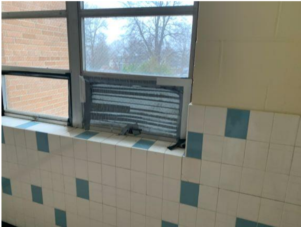
Photo 6 – Interior of Mother Teresa School Building. Stairwell window
