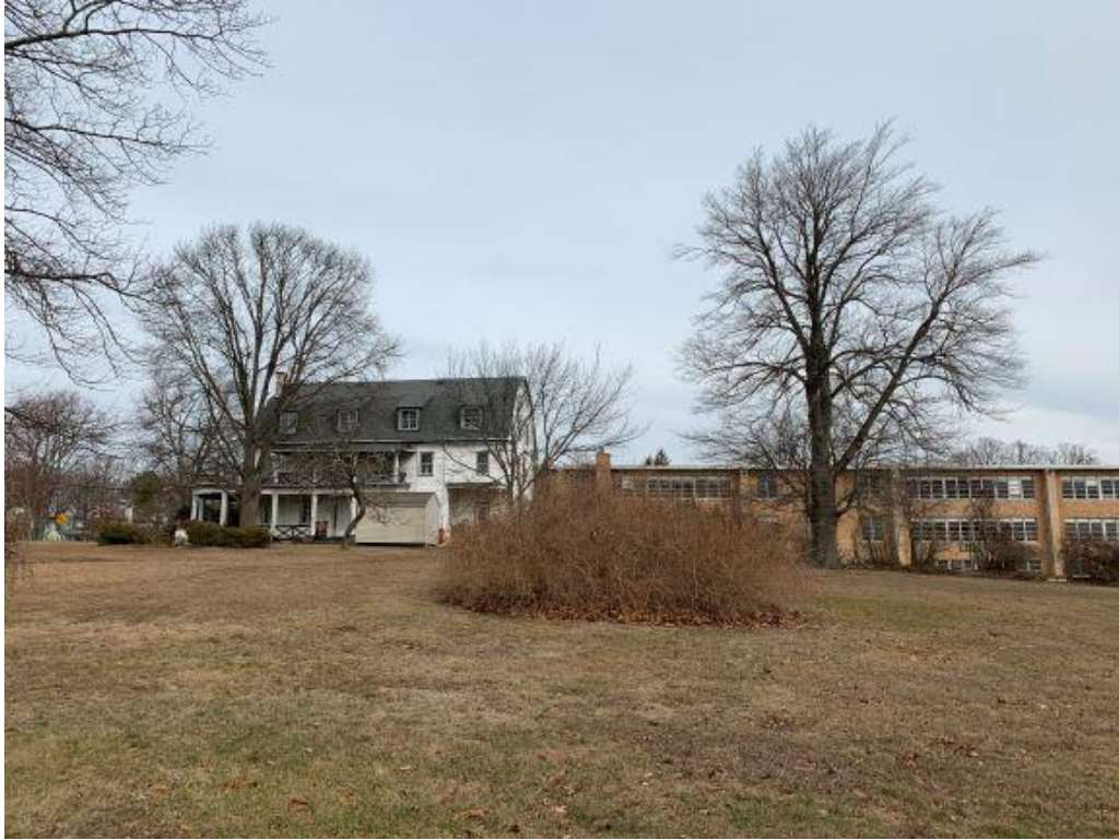
Photo 11 – Rear of School building and St. Agnes Thrift Shop. Photo taken from West Highland Avenue
