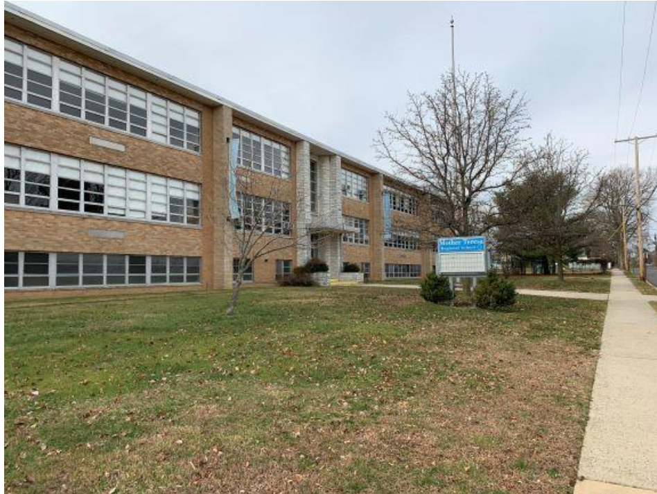
Photo 3 – Mother Teresa School Building. Photo taken from South Avenue
