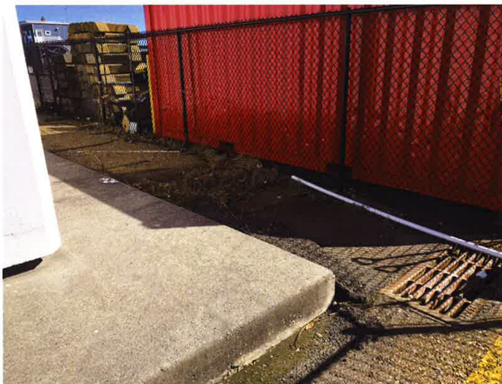
Photo 4: Storm Drain situated near tank Vaults
