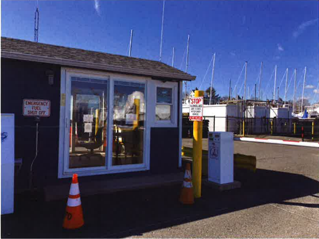
Photo 7: Emergency Shut Off located on Security Booth
