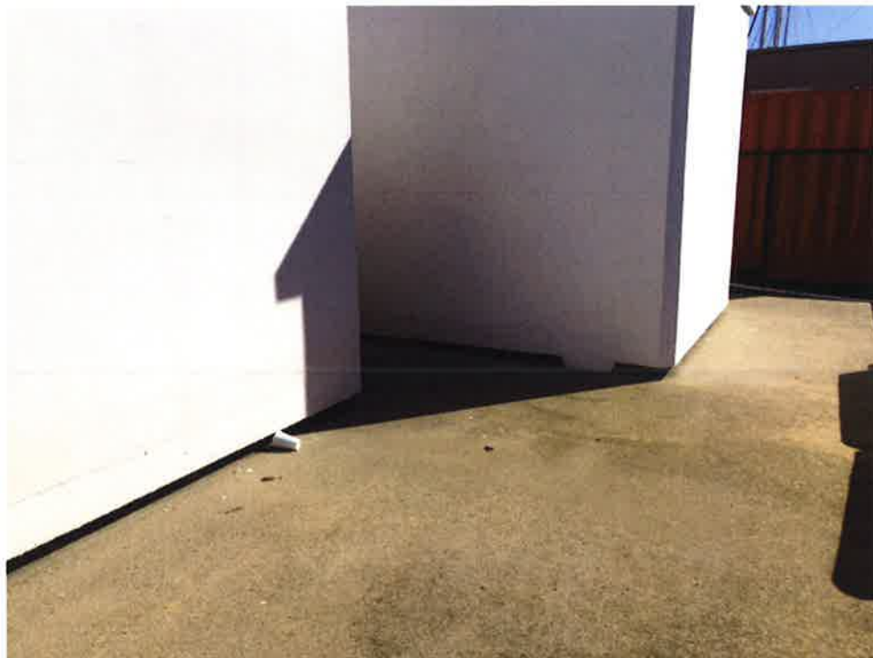
Photo 3: Motor Fuel Tank in Vaults situated on concrete pads
