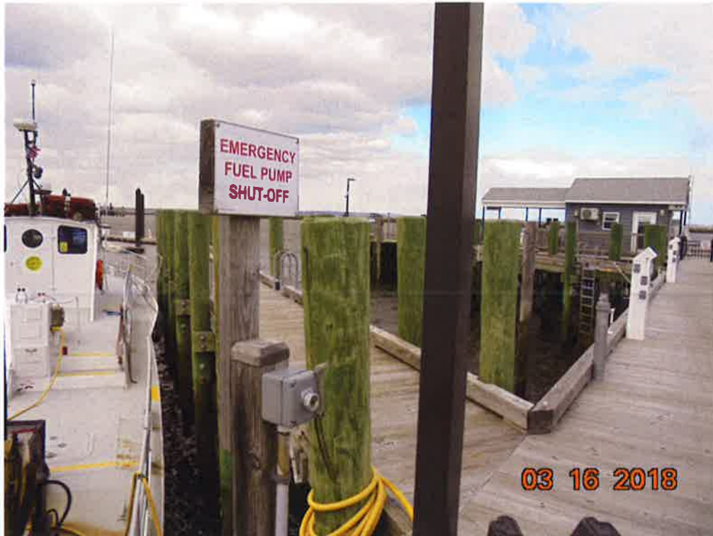
Photo 19: Emergency Shut Off for Dock Dispensers
