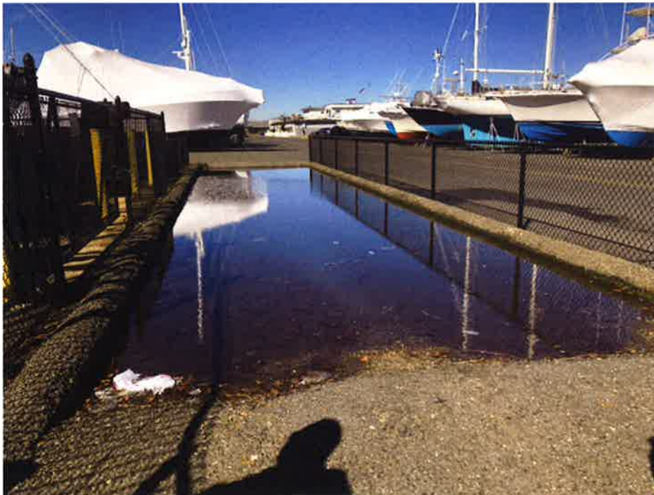
Photo 2: Containment area for fuel delivery trucks
